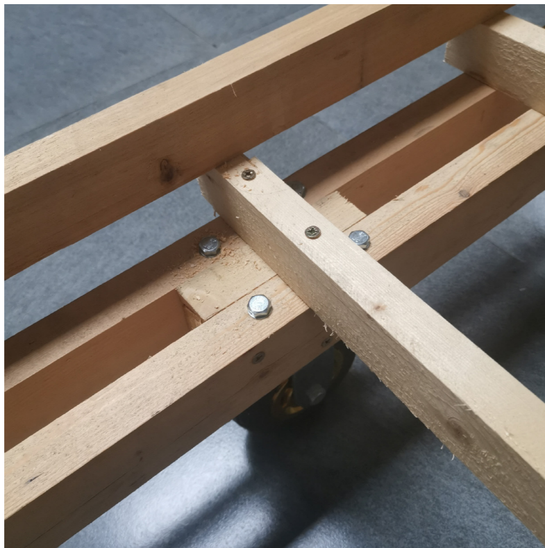
Continuous Beams and Connection Details
